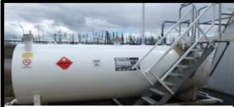
Ensure storage tanks have proper permits by authority having jurisdiction under the fire code
